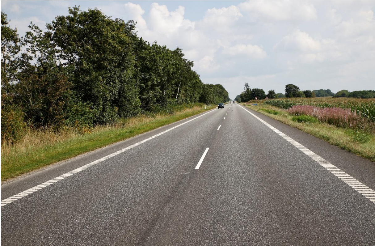
Figure 4. The road used for the Danish test site. (Photo: Trond Cato Johansen, Ramboll).
