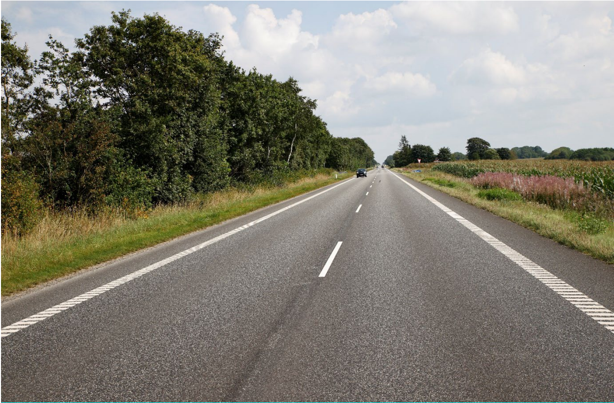
Figure 4. The road used for the Danish test site. (Photo: Trond Cato Johansen, Ramboll).
