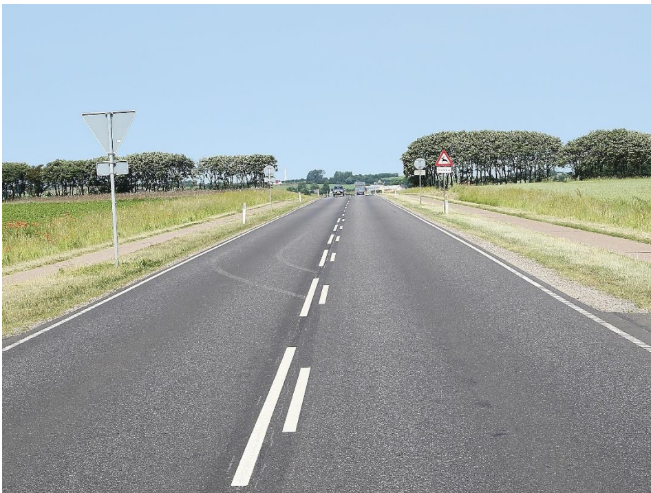
Figure 3. The road used for the Danish test site in Gørlev. (Photo: Trond Cato Johansen, Ramboll).
