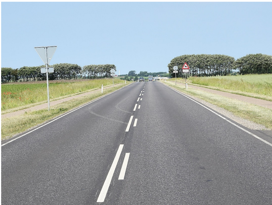
Figure 3. The road used for the Danish test site in Gørlev (photo: Trond Cato Johansen, Ramboll).
