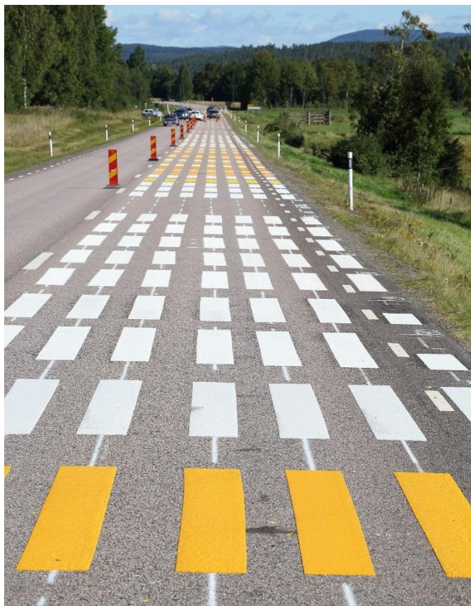
Figure 1. The test site in Sweden at the time of application in 2015. Photo: Trond Cato Johansen.
